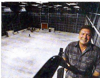
The Cape Town Film Studio accommodates sound studios, workshops and production offices
